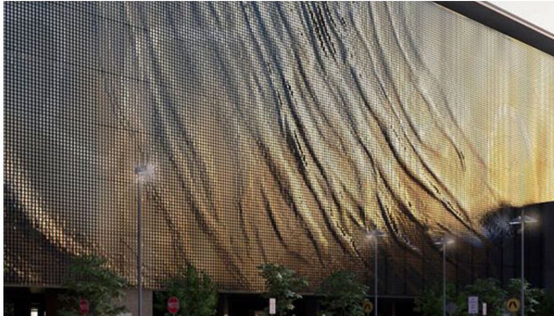
Figure 79: Ned Kahn facade https://nedkahn.com/portfolio-category/wind
