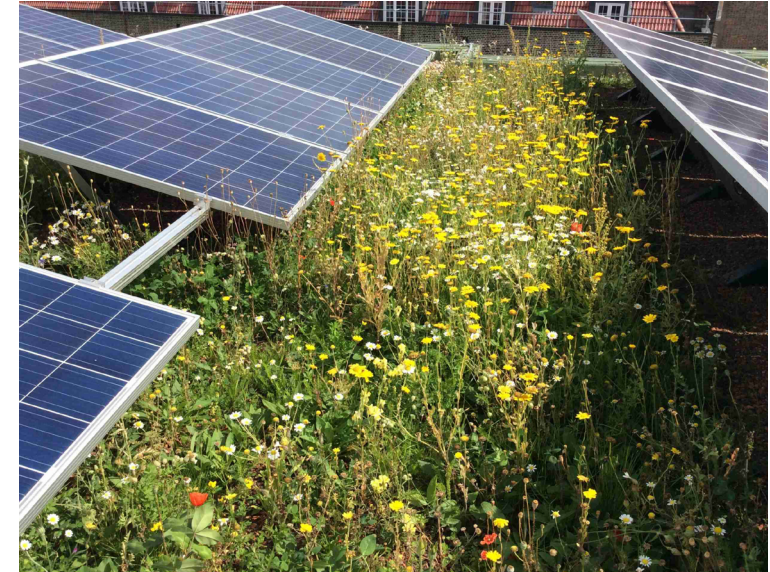
Figure 92: Green roof with solar panels Own image
