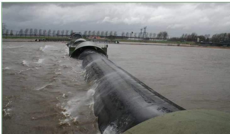
Figure 17: Inflatable dam, the "balgstuw" at Ramspol, the Netherlands.
