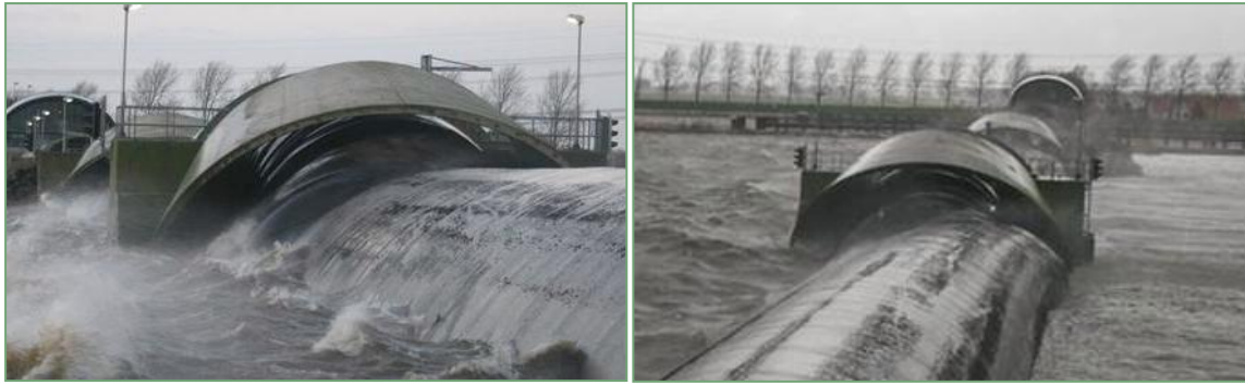
Figure 28: Folding and shifting of the “balgstuw” at Ramspol. (High water on the left side.)
