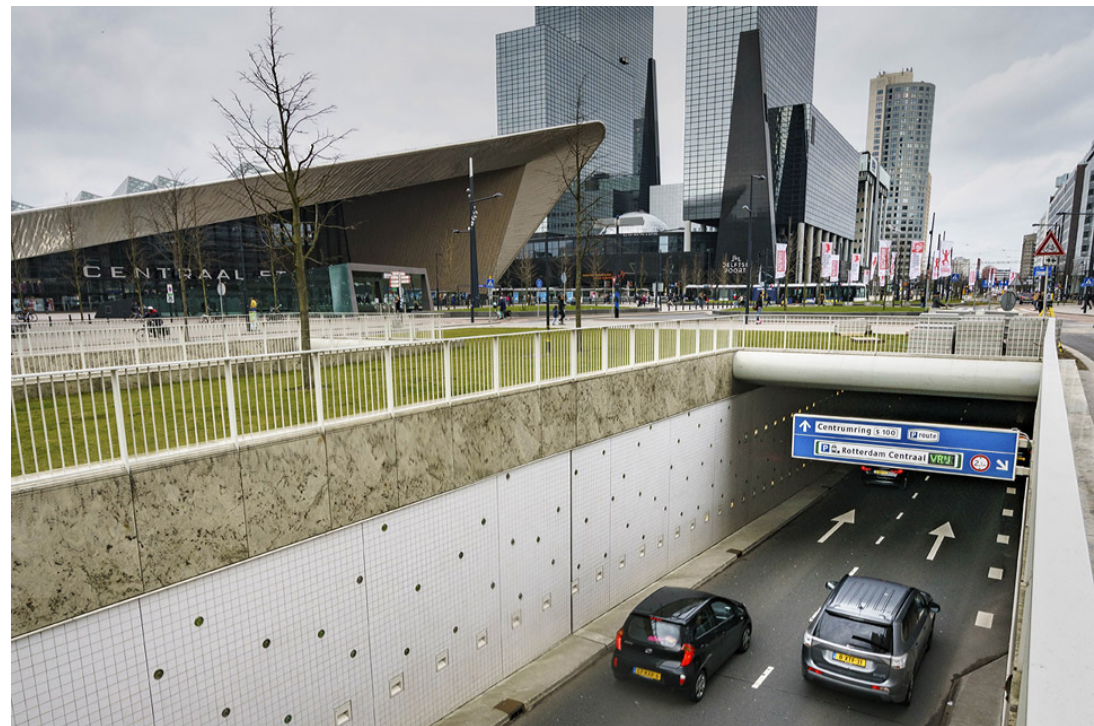
Figure 10: At Rotterdam central station, cars go underground to create more space for other traffic (OVMagazine, n.d.)
