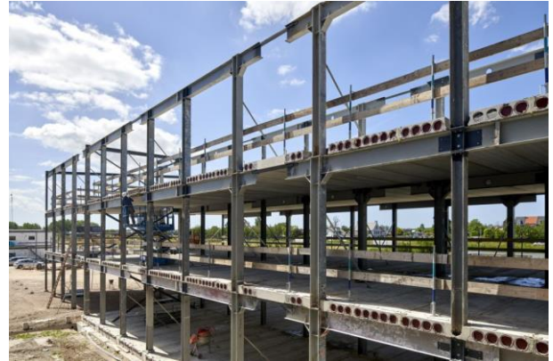
Figure 4: Use of donor skeleton on a large scale for Biopartner in Oegstgeest (The Netherlands) (source IMd/ Rene de Wit)
