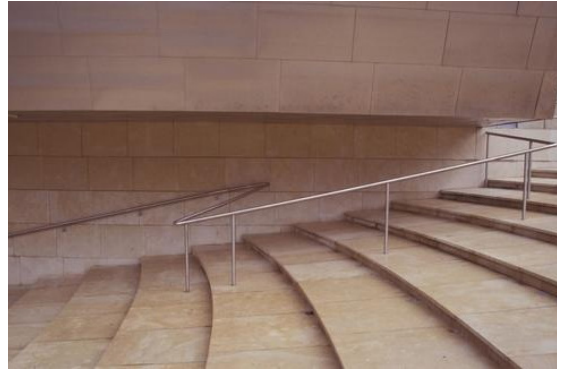
Fig. 28: Guggenheim, Bilbao Entrance area - iconic architecture creating disfunctional spaces
