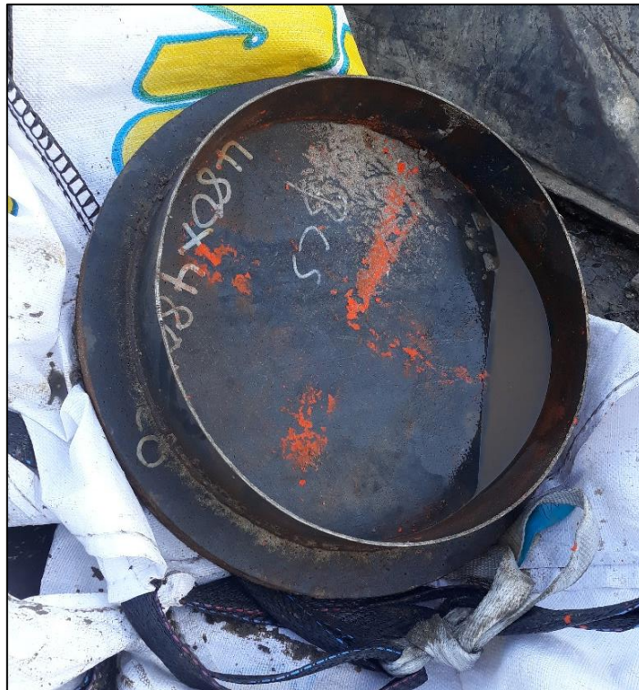
Figure 3.1: Sacrificial base plate used for the installation of the vibro piles
