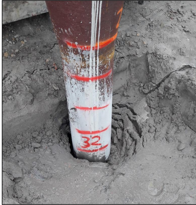
Figure C.3: Annular space around the auxiliary pile during pile driving
