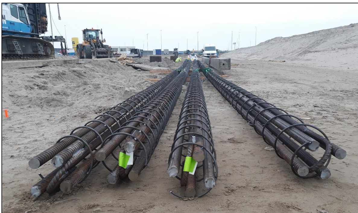
Figure 3.2: Steel reinforcing of the vibro piles lying on site in advance of instrumentation and installation
