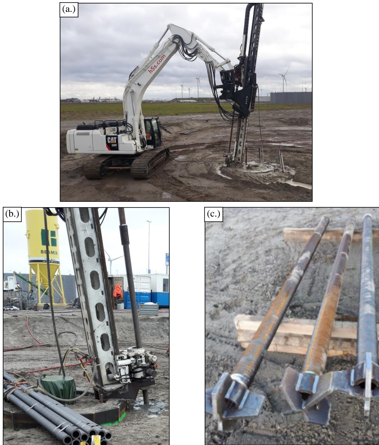
Figure 4.5: (a.) Installation of the grout anchors around the test pile (b.) Close up of the installation process, highlighting the use of the anchor guide frame in order to install the anchors at the correct position (c.) screw tip of the grout anchors (photo: Gust van Lysebetten, WTCB)
