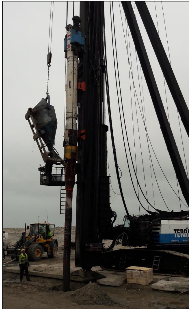
Figure C.5: Concrete replenishment during the withdrawal of the auxiliary tube
