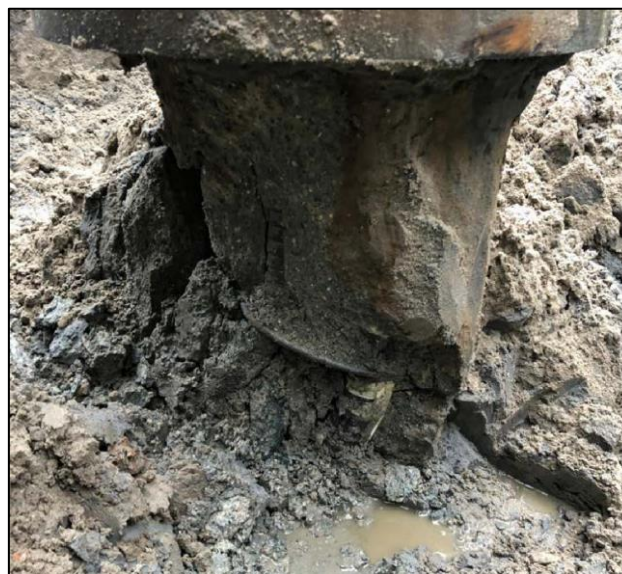
Figure 5.13: Close-up photo of the breakage immediately underneath the sleeve of pile P03 (Photo credit: Gust van Lysebetten, WTCB)
