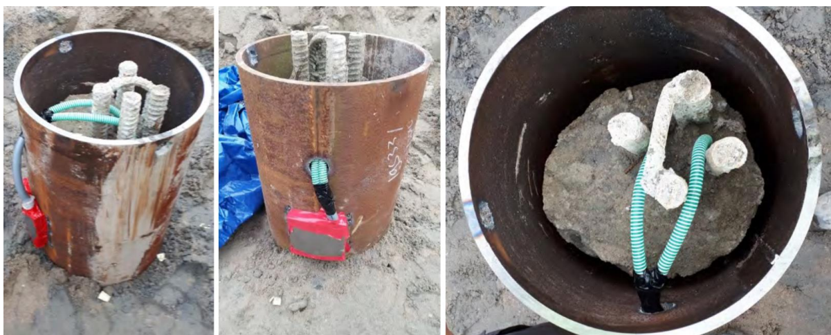
Figure 3.5: Vibro pile after the installation of the two metre sleeve around the uppermost part of the pile shaft without grout (Photos: Gust van Lysebetten, WTCB)
