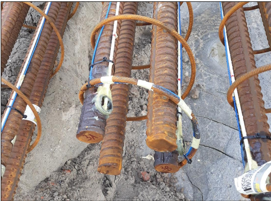
Figure 4.10: Close-up of the base of the reinforcement cage. Note the loop in the BOFDA cable (blue cable) across the spiral reinforcing. The FBG cable (white) terminates at the end of the reinforcement cage
