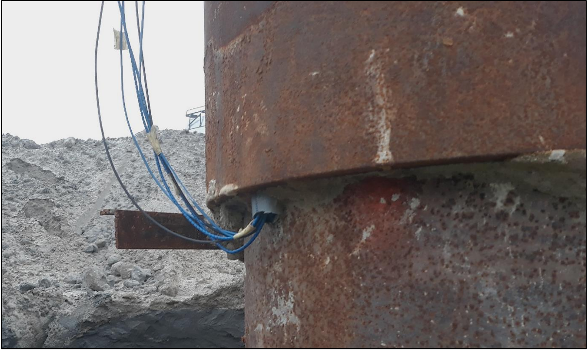
Figure 4.11: Egress point for the fibre optics between the pile cap and pile sleeve. Grout was used to fill the annular space between the pile cap and pile sleeve, with a PVC facilitating the safe passage of the fibre optics through the annular space
