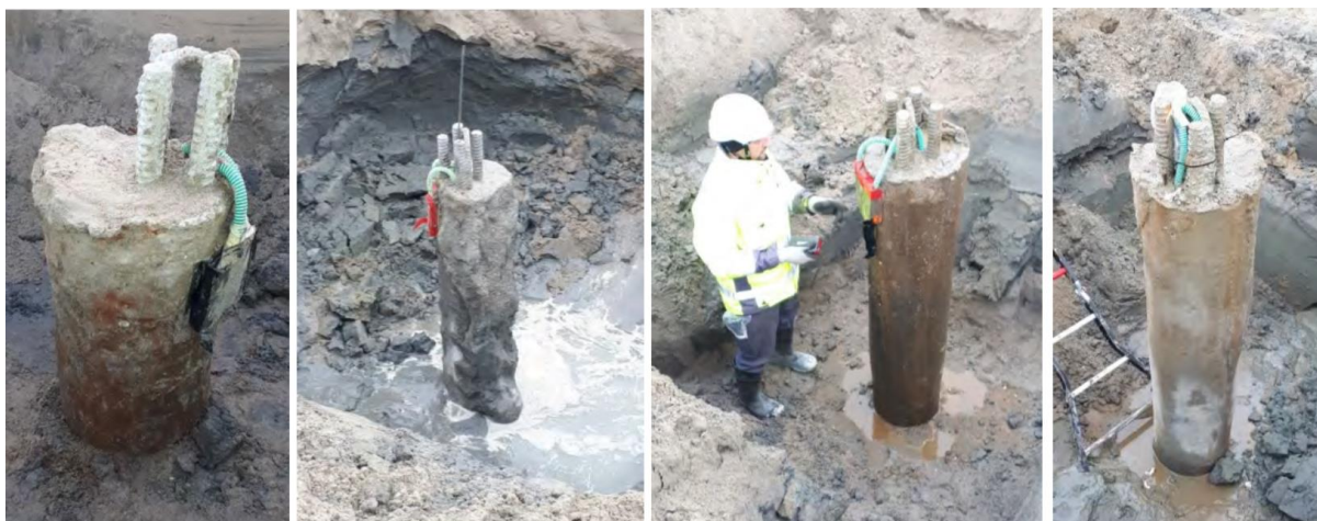
Figure 3.4: Pile heads of the four vibro piles immediately after installation. Note the non-centric placement of some of the reinforcement (Photos: Gust van Lysebetten, WTCB)
