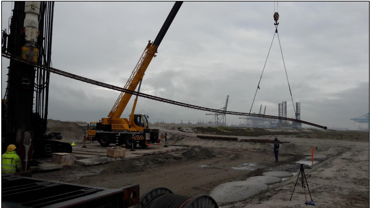
Figure C.4: Lifting of the reinforcement cage for P11 using a mobile crane and the drilling rig crane (left)
