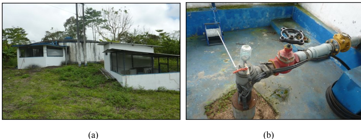
Figure 3.5- (a) Storage tank and pumping station and (b) extraction pump at Bellavista
