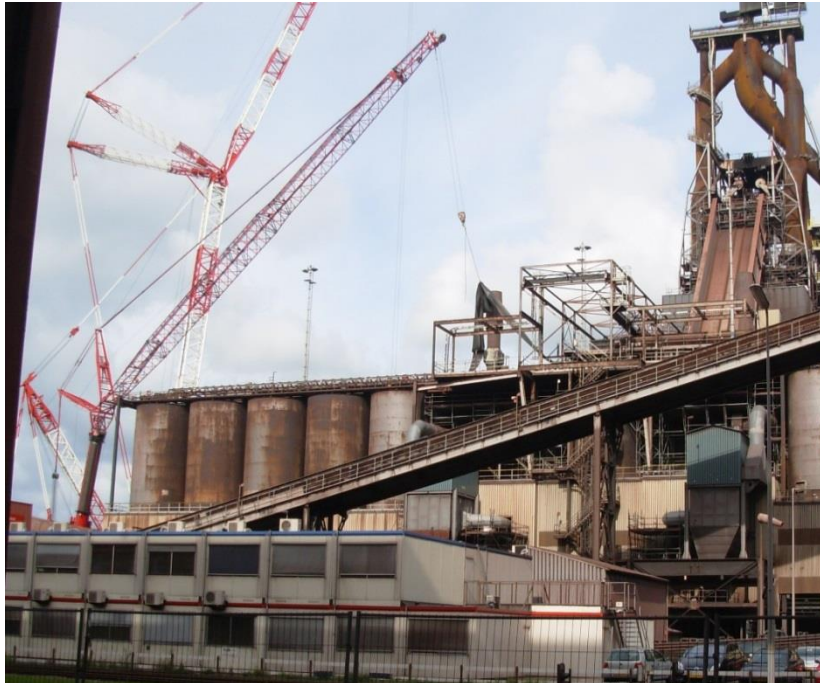
Figure 13: A crane is required to replace the belt
