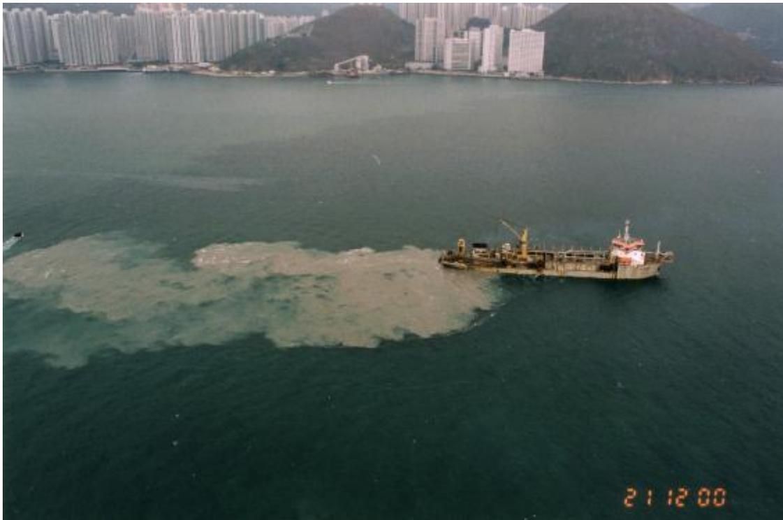
Figure 1.1: Picture of an overflow plume in practice
