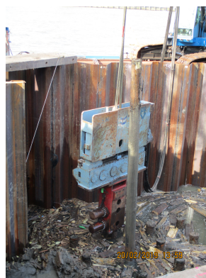
Figure 5.3: Maaskade strip. Removal of timber floor (left) and removal of timber piles (right). Pictures provided by the Port of Rotterdam.
