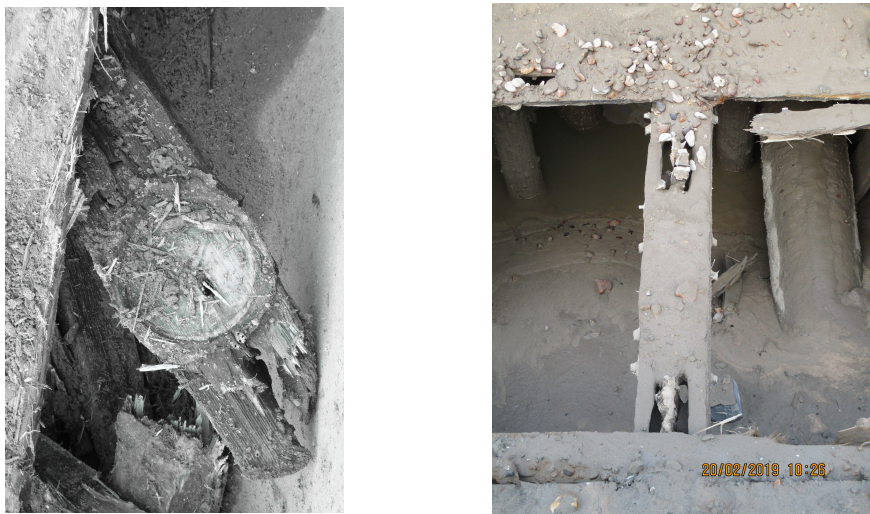
Figure 5.7: State of softwood. Left: clearly visible connection places are less deteriorated. Right: Bad state of mortise and tenon joints.
