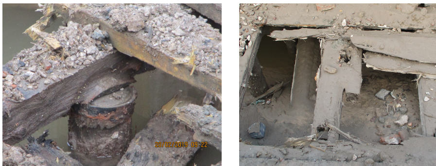
Figure 5.11: Eccentricities in placement of the beams on the pileheads. On the right even a much wider beam had to be placed to accommodate the poor pile placement
