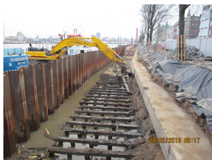
Figure 5.3: Maaskade strip. Removal of timber floor (left) and removal of timber piles (right). Pictures provided by the Port of Rotterdam.
