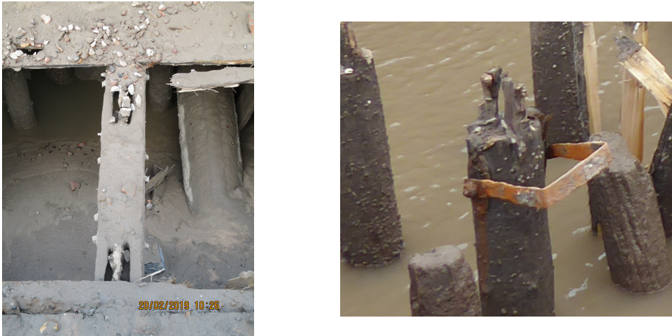
Figure 6.11: Left: Standard Mortise and Tenon joint (e.g. pile row 3). Right: Braced Mortise and Tenon joint (e.g. pile row 2).
