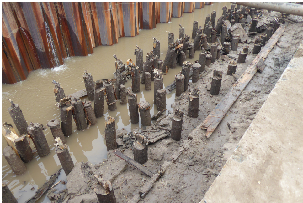
Figure 4.18: Start of section 4-1 from the site investigation in 2019. Note the large amount of piles due to overlap of structure in the 2nd and 3rd beam row. It may be possible as well that these piles are even older piles (from the 1875 wall), as the piles from nearby wall section 3-1 are not as high, though sectional drawings of section 7-1 suggest differently: the old wall is behind the quay with relieving platform.
