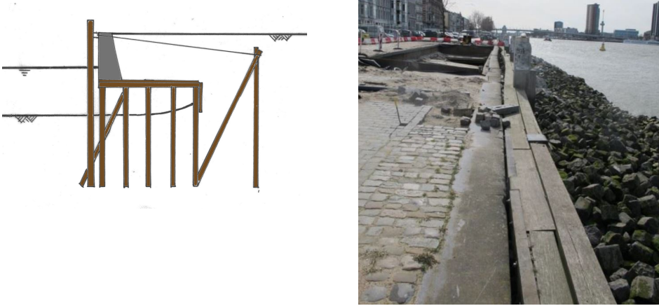
Figure 1.1: A quay wall with relieving platform (left), inspection of the failure of the Maaskade (right) [6] .
