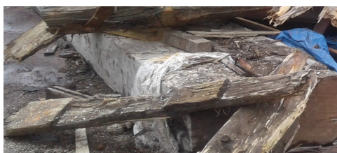
Figure 5.7: State of softwood. Left: clearly visible connection places are less deteriorated. Right: Bad state of mortise and tenon joints.
