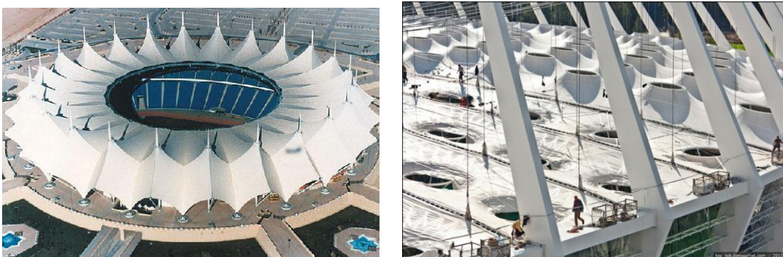
Figure 7-5 Single layer double curvature roof structures. Left: King Fahd stadium Right: Kiev Olympic stadium (Source: www.stadiumdb.com )
