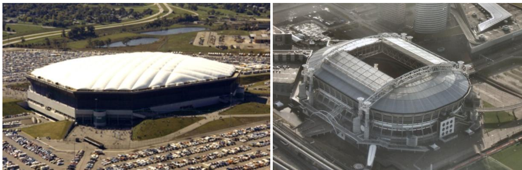
Figure 4-17 Left: Permanent playing field roof cover (Silverdome stadium) Right: Temporary playing field roof cover (Amsterdam Arena). Source: www.stadiumdb.com
