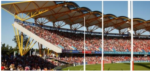
Figure 7-8 Single curved post-tensioned roof structure Mettricon stadium (Source: www.stadiumdb.com )
