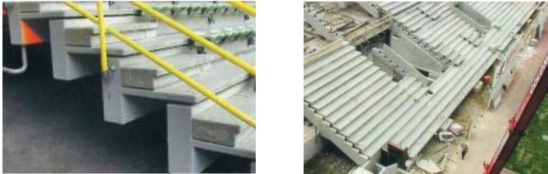
Figure 6-5 Left: Tilted t-profile , Right: Z-profile Dortmund Energie stadion Cologne Source: (Nixdorf, 2007)
