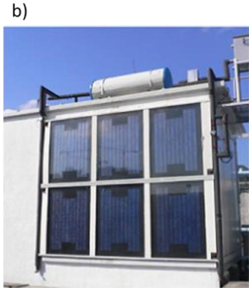
Figure 2-7a) BIPV/T with air. It is a combination of PV modules and a transpired collector [24]. b) BIPV/T with water. Solar collectors on façade combined with PV modules [25]
