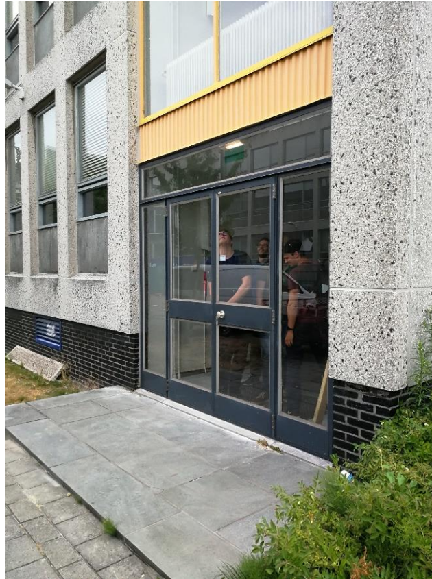
Figure 9. An emergency exits was close during the evacuation exercise
