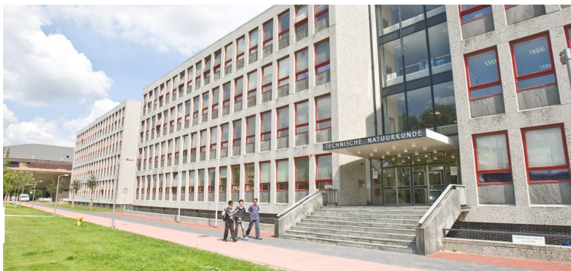
Figure 5. 3D model for Faculty of Applied Sciences (upper) and real picture of the entrance (bottom) (2016)
