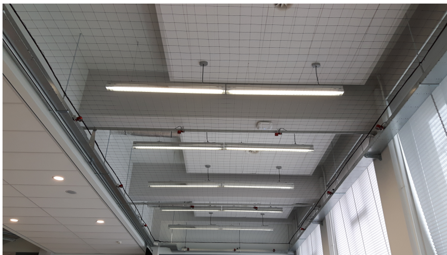
Figure 3-4: Gutter around the lab perimeter with mounted cameras
