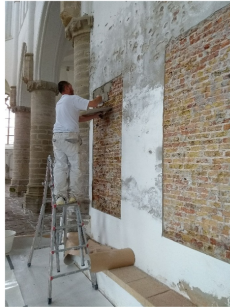
Fig. 1. Left: Plan of the church with indication of the location of the test area; Right: application of the plaster on the test area.
