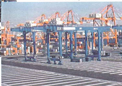
Wan-Hai Line, Tokyo Manned Trucks and automated cantilever RMGs with automated crane and trolley movements
