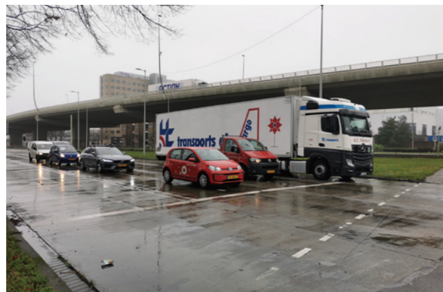
Fig. 6.2.4. Highway in Nieuw-West. Photographed by author.
