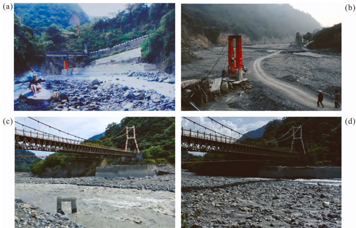
Fig. 1. Risk to infrastructure due to river bed elevation change, as illustrated by the Laonong River at the Aqiba bridge site: (a) before 2009 (roadside hot spring advertisement); (b) in February 2010, after the Morakot geomorphic flood; (c) in September 2019; (d) in August 2021 (see text for description).
