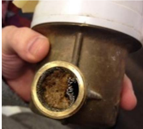
Figure 10: clogged water meter
