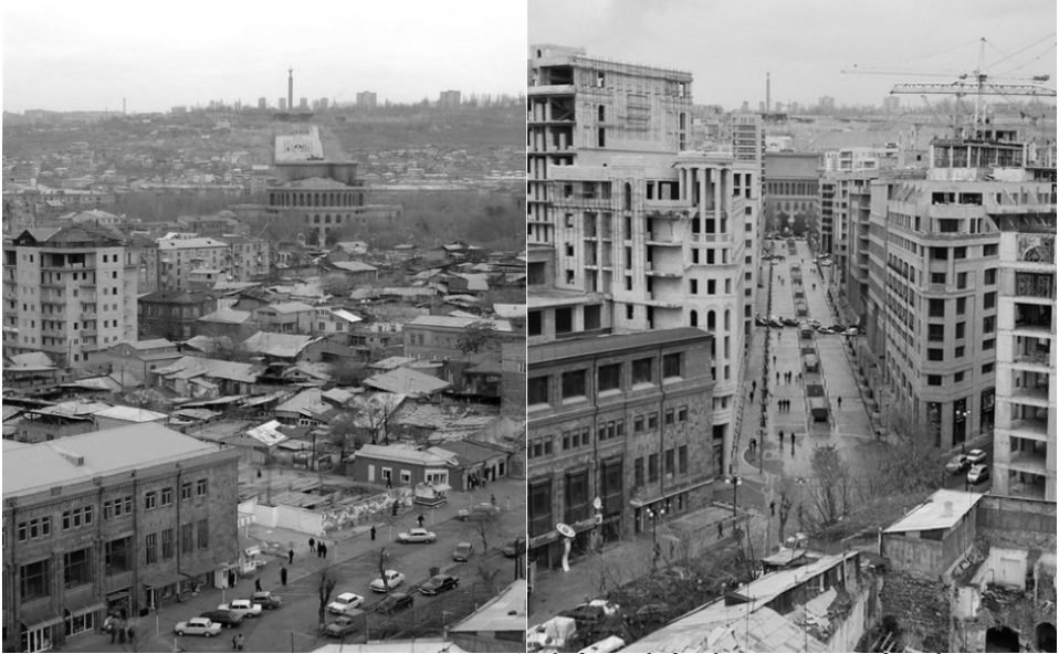
19. Site before and after the construction of Northern Avenue
