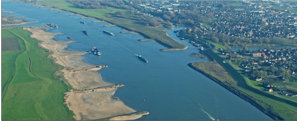
Figure 4.12: Floodplains and dikes along the Waal during deepening of 'kribben' by Van Oord (2012).
