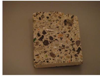
(b) Concrete blocks made from the BA aggregate.
