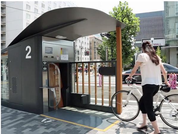
Figure 7-1: Underground bicycle storage 5
