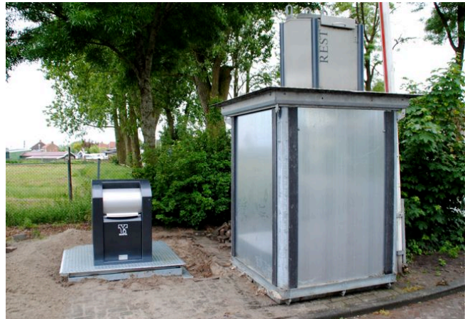
Figure 7-2: Underground disposal containers 6
