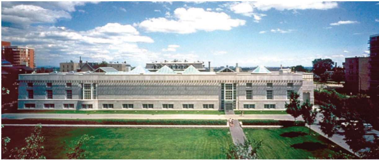
Figure 6: Exterior of the CCA, north facade (Peter Rose + Partners, n.d.)
