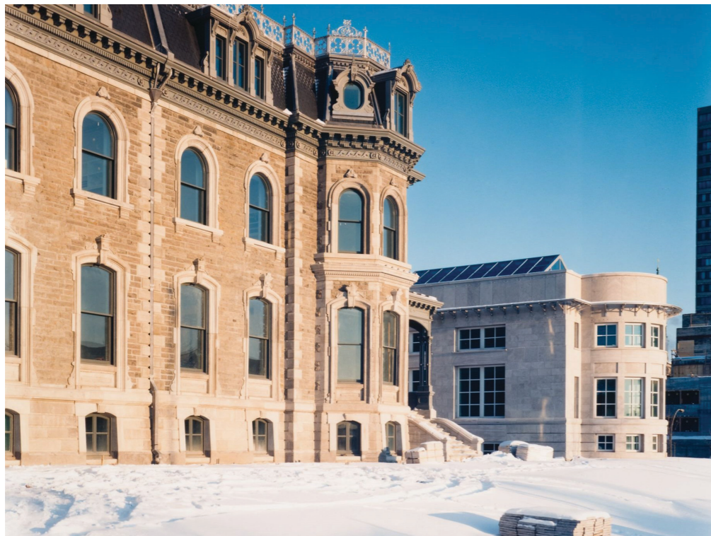
Figure 1: View of the south elevation showing Shaughnessy House and Scholars' Wing (Gabor Szilasi, 1989)
