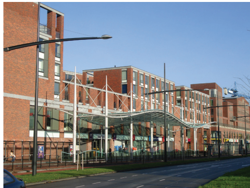
Tram/bus station Delft, 2008, Mick Eekhout
