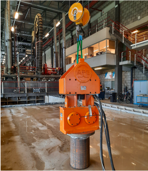
Fig. 6. A close-up view of the pile, vibro-hammer and crane assembly, at the end of installation.
