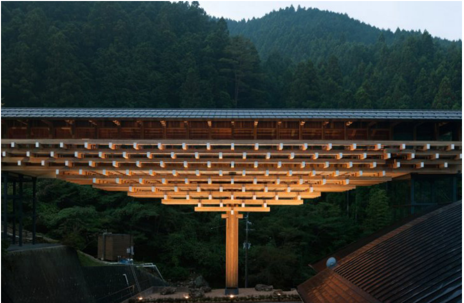
Figure 16 Detailed view of Bracket system Yusuhara bridge museum ( https://www.archdaily.com/199906/yusuhara-wooden-bridge-museum-kengo-kuma-associates )
