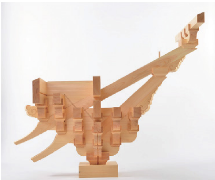
Figure 8 Bracket joinery detail from Traditional Japanese wood joinery and its modern translations , by F. Horace, 2024.
