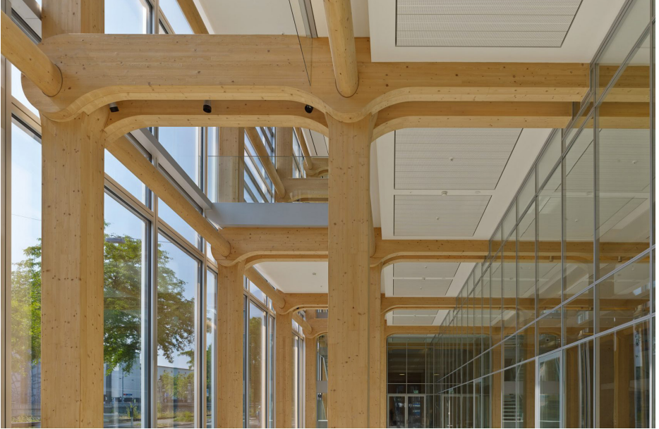
Figure 20 Interior structure Tamedia office building ( https://www.archdaily.com/478633/tamedia-office-building-shigeru-ban-architects )
