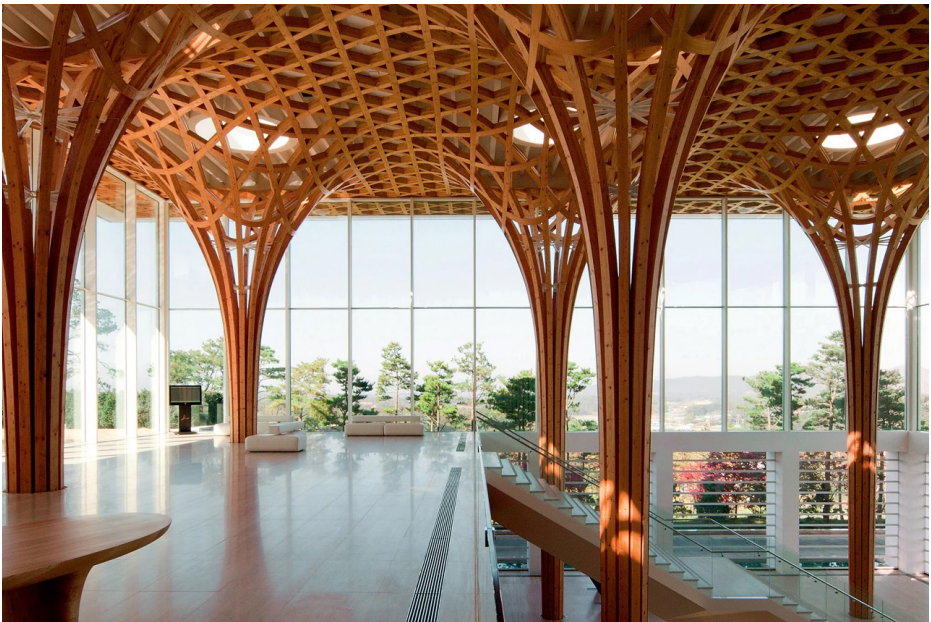
Figure 13 Vertical column transition into the ceiling grid at the Haesley Nine Bridges Clubhouse from Haesley Nine Bridges Golf Clubhouse, Yeosu - Shigeru Ban, by Architectura Viva, 2021, ( https://arquitecturaviva.com/works/club-de-golf-haesley-nine-bridges-0# ).
