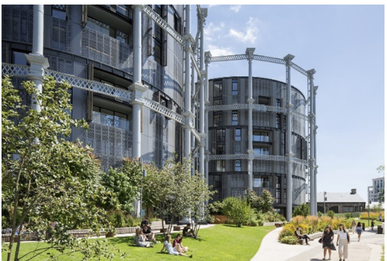
Fig. 4.6 The gasholders transformed into apartments. (left)
