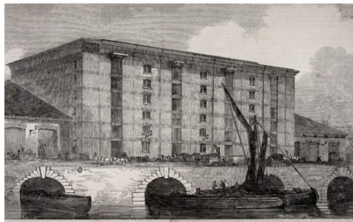
Fig. 1.11 The granary and the basin
