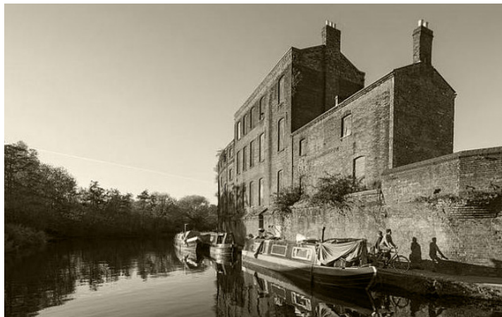
Fig. 1.10 Coal and Fish Offices
