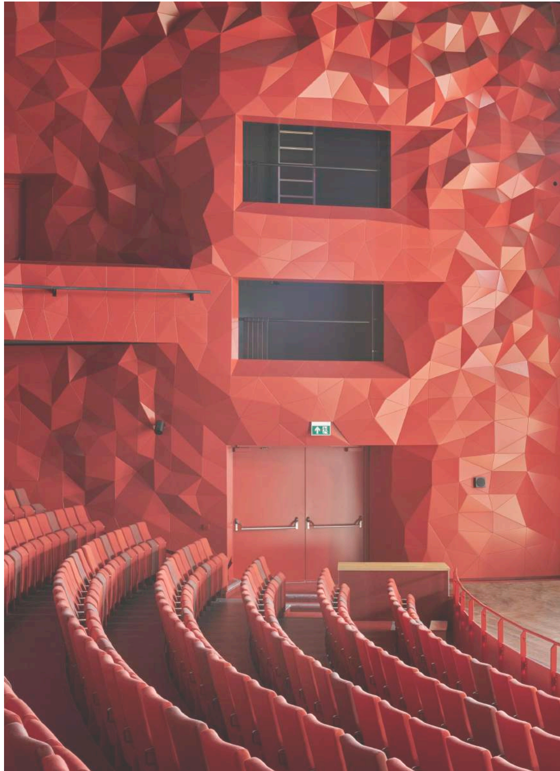
Figure 13. Internal Aluminium Cladding of Theatre Zuidplein Studio Rap, (n.d.)
