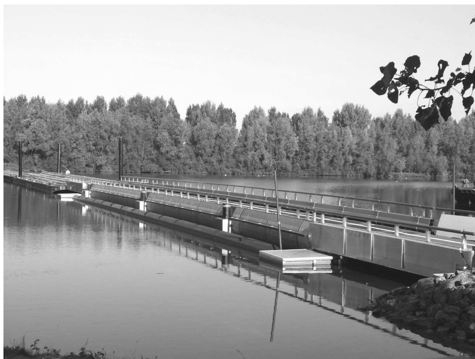
Figure 6.2 Floating road near Den Bosch (Ministerie van Verkeer en Waterstaat, 2004)
