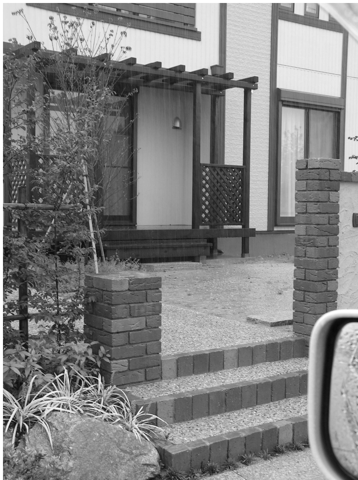
Figure 3.2 Reducing damage in case of flooding: high level difference between road level and floor level. (Source: Frans van de Ven)
