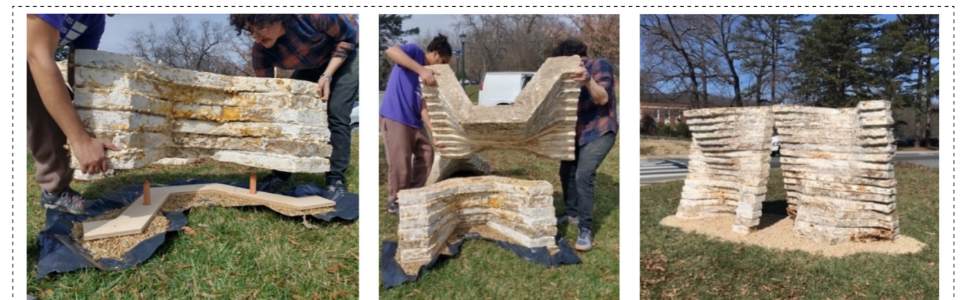
Figure 12: Installation of the prototype onsite (Source: Dessi-Olive 2022)
