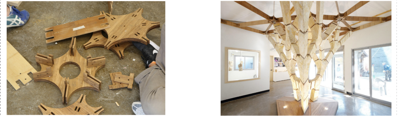
Figure 10: (left) Assembly of CNC-cut grid components through jointless, slit-and-slot connections and wooden dowels, (right) MycoTree is the centrepiece of the "Beyond Mining - Urban Growth" exhibition at the 2017 Seoul Biennale of Architecture and Urbanism in Korea. (Source: Heisel, 2017)
