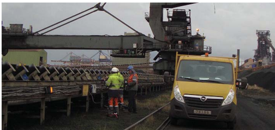
Figure 3: Idler rolls inspection
