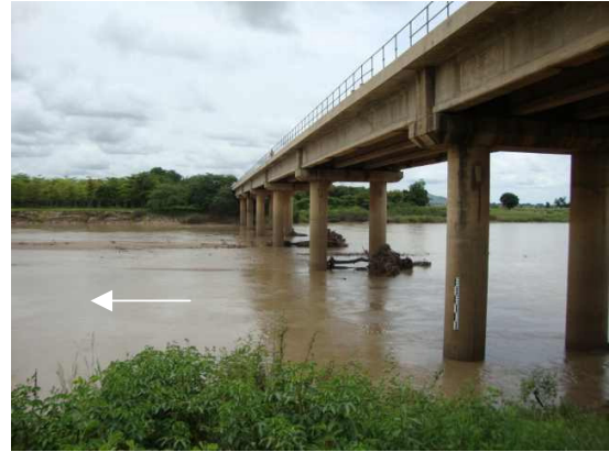
Figure B.12 Bridge over White Volta (Yarugu)
