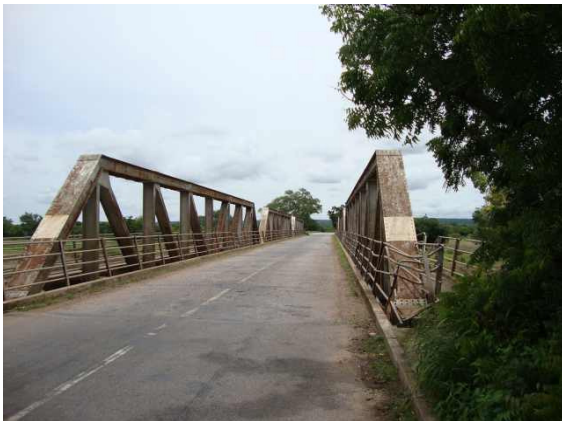
Figure B.3 Pwalugu bridge
