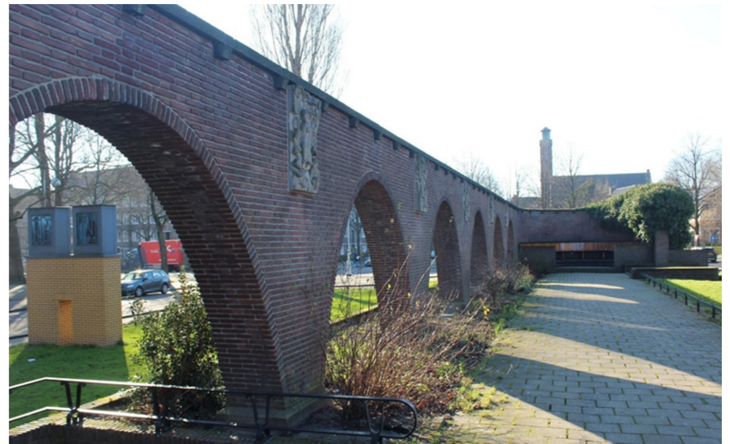
Figure 9: Wall with Arches, Semi-enclosed Seating and Later Added Pillars. (by author)
