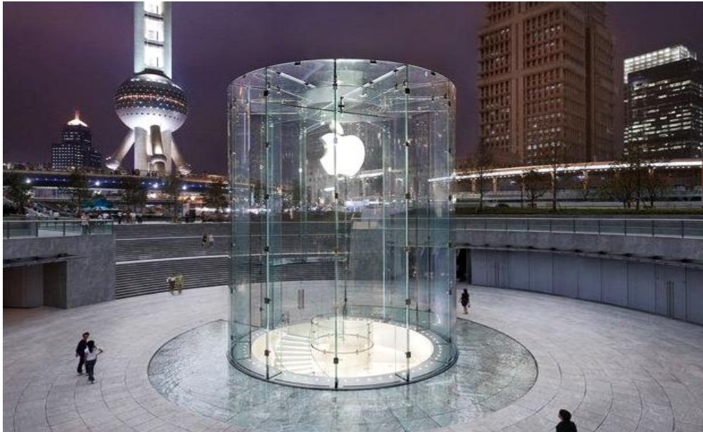
Figure 2.8: The figure above provides an external view of the 12.0 m-height glass cylinder of the Apple Store located in Shanghai, forming the entry to the store placed underground. The cylindrical structure is composed of 62 glass panels, 2.5 m wide and 12.5 m tall. The panels are 6-layers thick and are formed from tempered, ultra-clear, bubble-, strain- and scratch-free glazing (Source: Sivagnanasundram, 2011).
