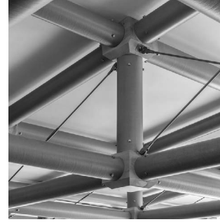
Shigeru Ban Architects. (2013). Madrid paper pavilion . https://shigerubanarchitects.com/works/exhibitions/madrid-paper-pavilion/
