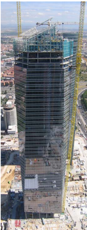
Figure 4.3-1: Torre de Cristal under construction
