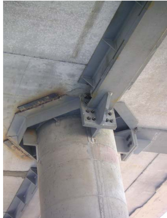
Figure 5.3-3: Column-beam connection
