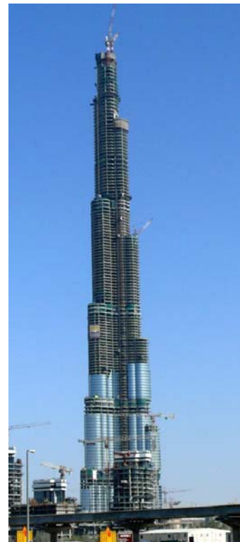
Figure 2.1-18: Burj Dubai under construction [40]
