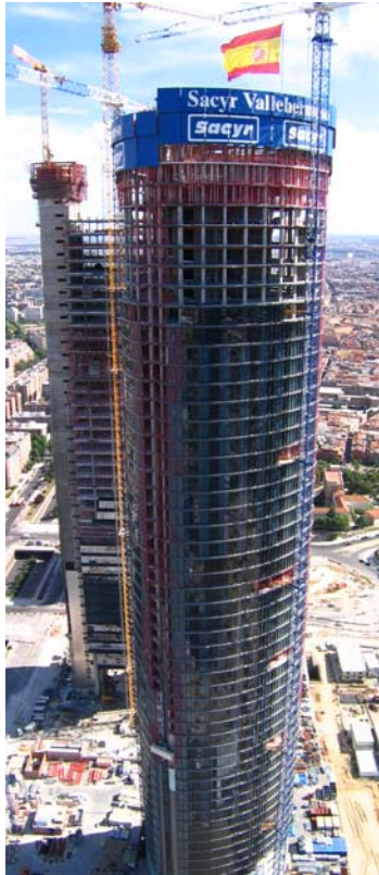
Figure 4.4-1: Torre Sacyr Vallehermoso under construction
