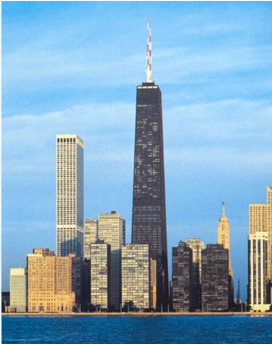
Figure 2.1-10: John Hancock Center in Chicago [9]
