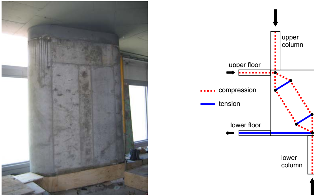
Figure 5.2-2: Concrete transition block with strut-and-tie model
