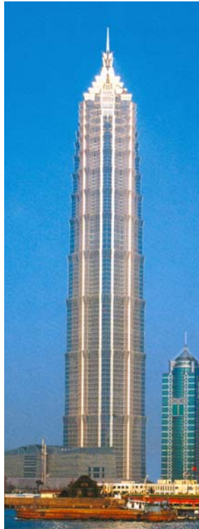
Figure 2.1-13: Jin Mao Tower in Shanghai [9]
