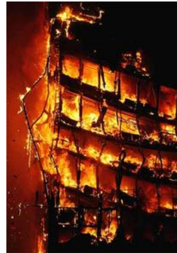
Figure 2.2-4: Fire in Torre Windsor in Madrid [17]
