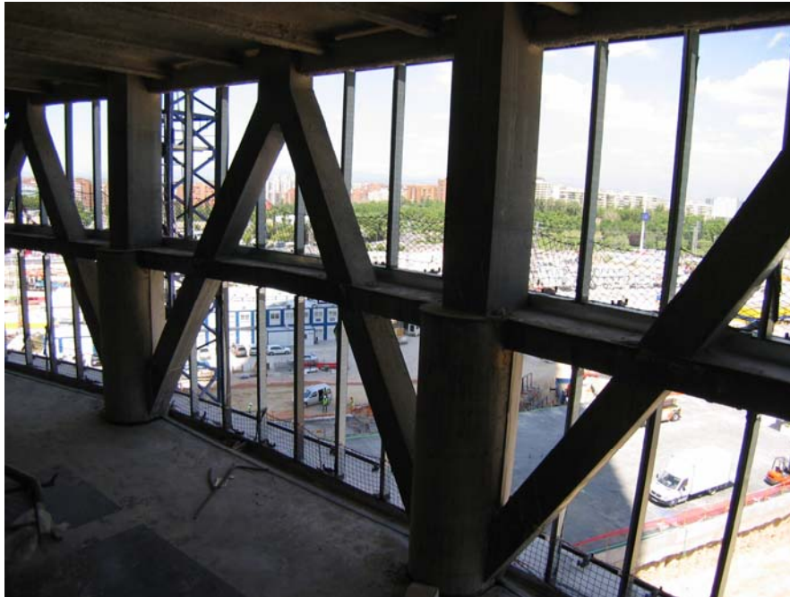
Figure 5.4-6: Outer transfer truss
