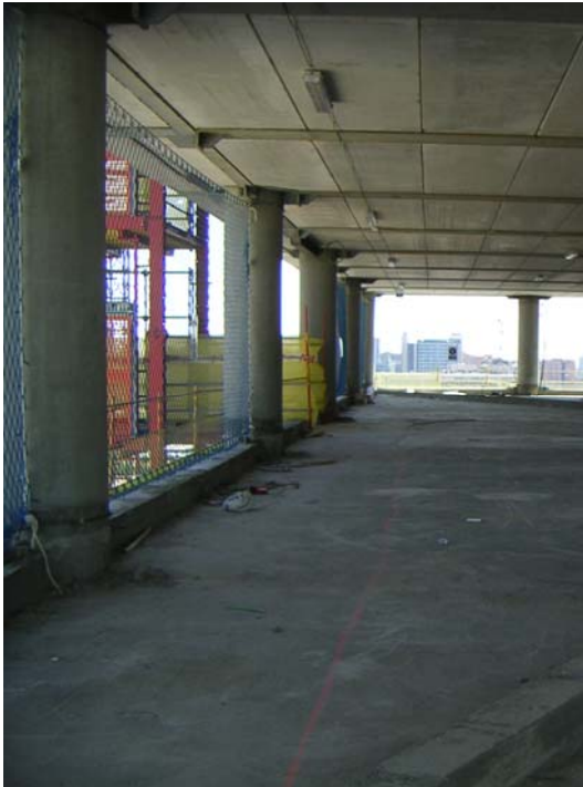
Figure 5.3-2: Integrated floor beams
