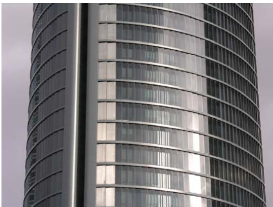
Figure 4.4-3: Fish-scale outer façade
