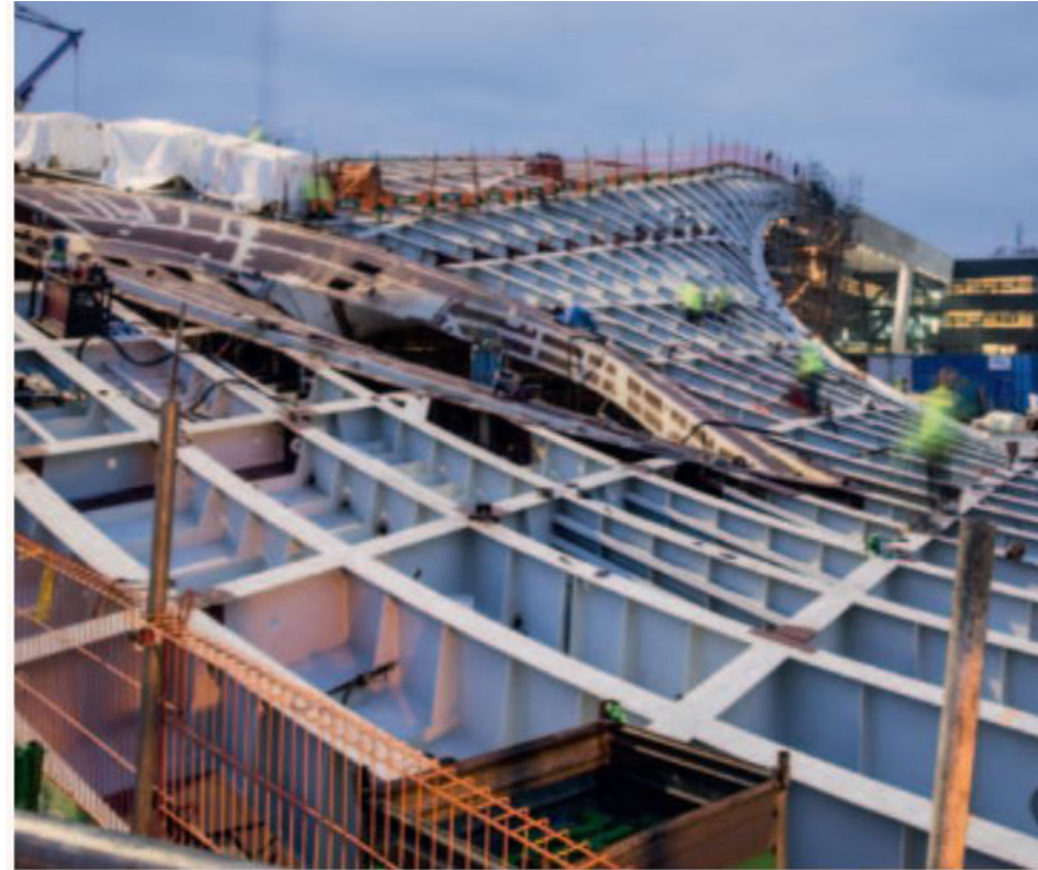
Arnhem Central - UNstudio Reversed boat construction
