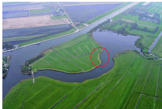
Figure 2-1: Aerial photograph of the Leendert de Boerspolder. The location of the dyke which was tested is highlighted in red
