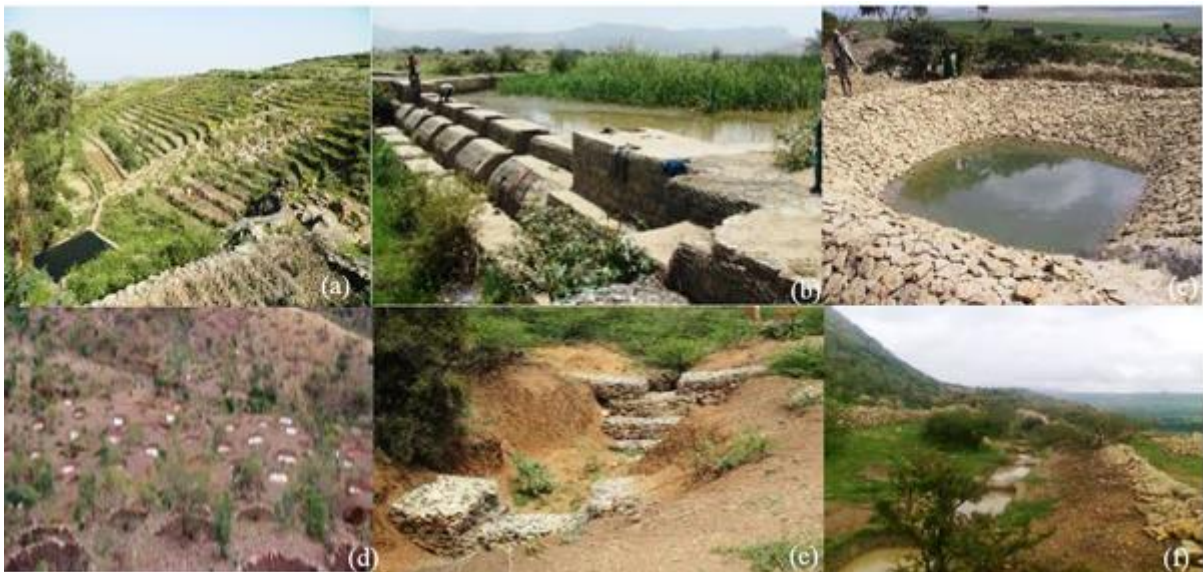
Figure 7.2: Physical SWC interventions in the Geba catchment of the Upper Tekeze headwaters: (a) terraces, (b) check dams, (c) water harvesting structures, (d) percolation ponds at the top of hills, (e) gully rehabilitation using gabion, (e) deep trenches at the bottom of hills (sources: (Woldearegay K & Tamene L, 2017; Yosef & Asmamaw, 2015).
