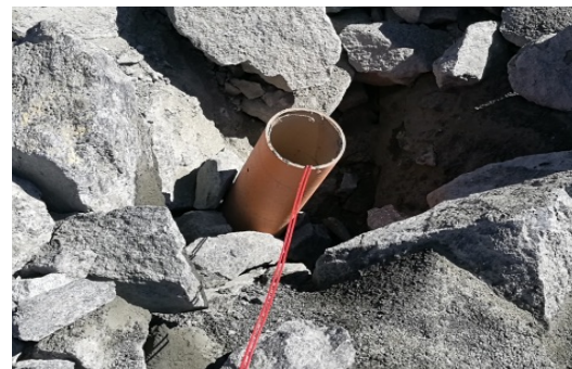
FIGURE 22: CARTBOARD PROTECTION OF DRILLHOLES
