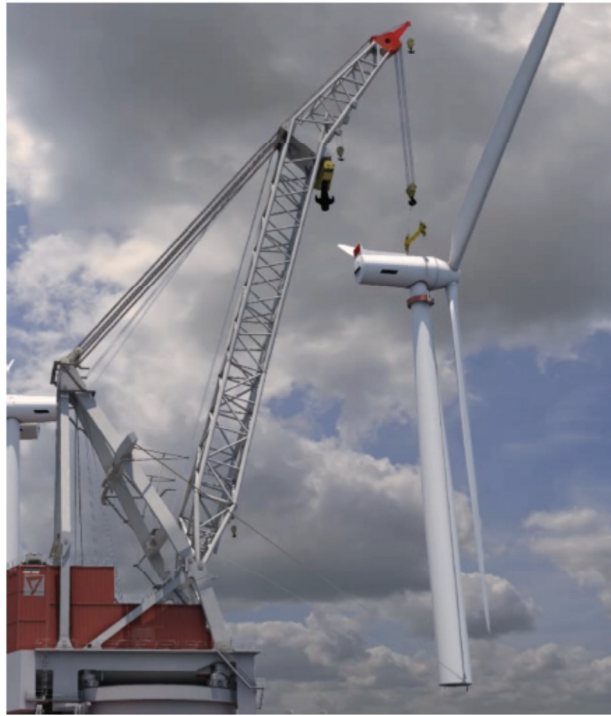
FIGURE 2-5: IMPRESSION OF OLEG STRASHNOV MAKING A SINGLE LIFT. SOURCE: SHL
