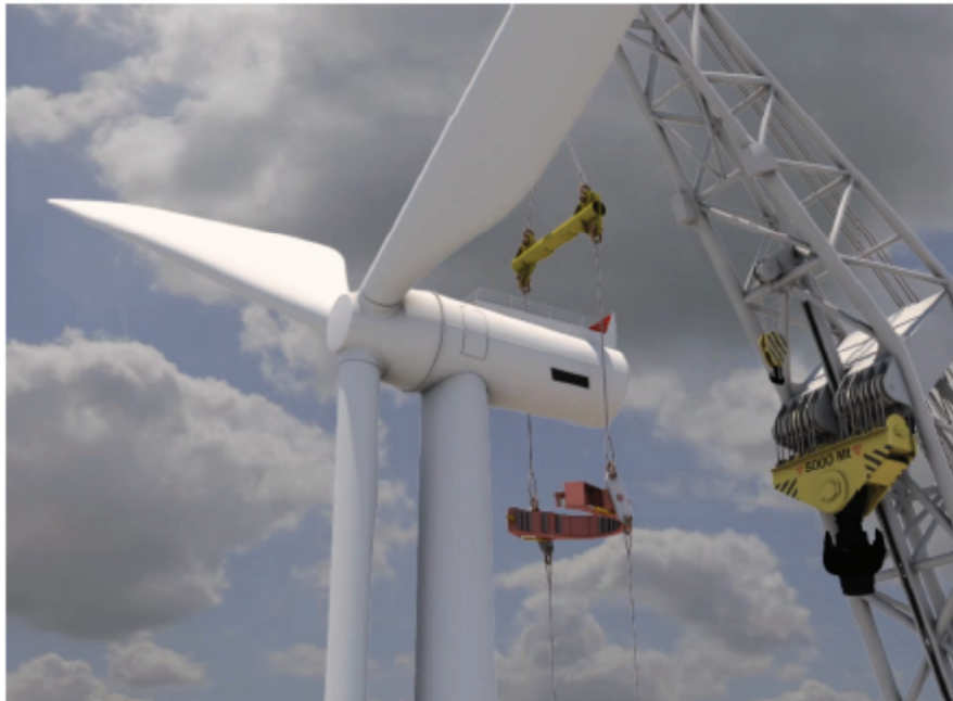
FIGURE 2-6: RIGGING ARRANGEMENT ENVISIONED FOR SINGLE LIFT. SOURCE: SHL
