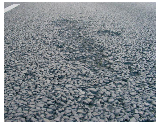
Figure 6: the decisive damage form in double layer porous asphalt; ravelling of asphalt
