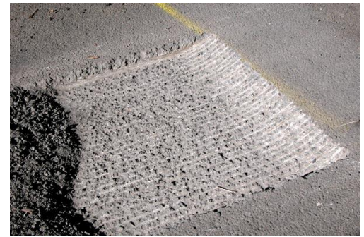
Figure 1: first step of resurfacing of pavement; milling-out old top layer
