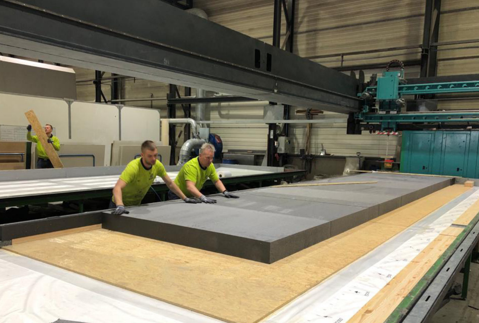
Figure 23 RC Panels Factory - Panel manufacturing (picture by the author)
