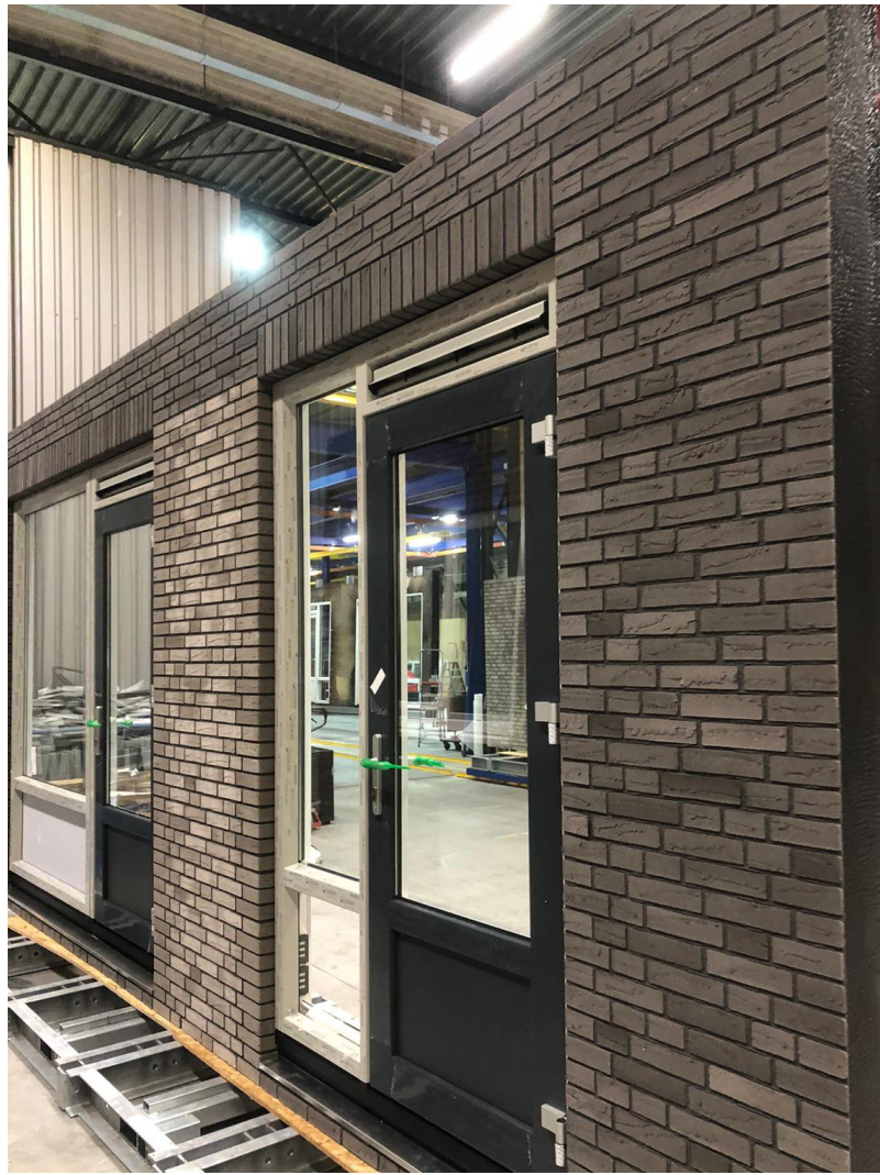
Figure 26 Finished facade waiting to be transported to the final destination (picture by the author)
