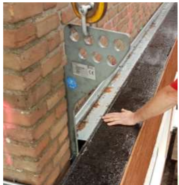
Figures 56 (top and bottom) 56 Facade Hoisting
