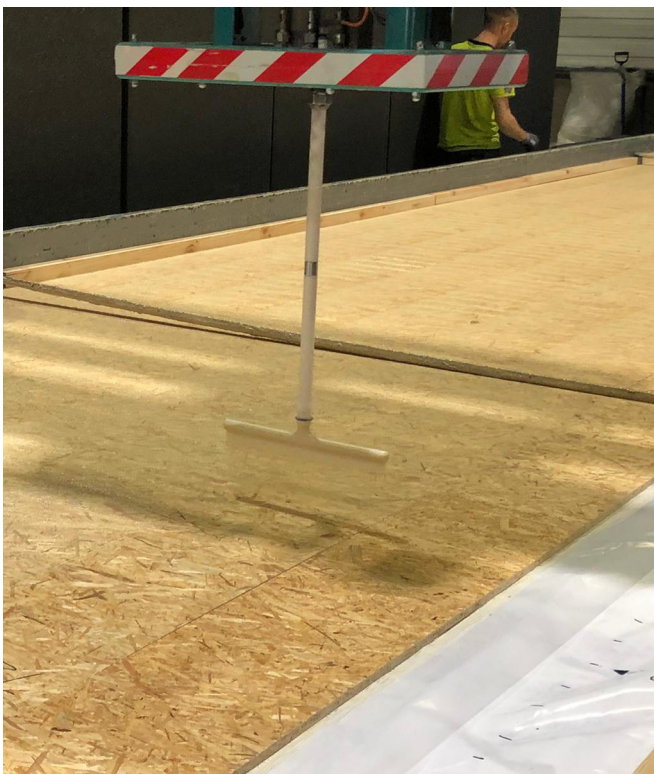
Figure 53 Polyurethane adhesive installation
