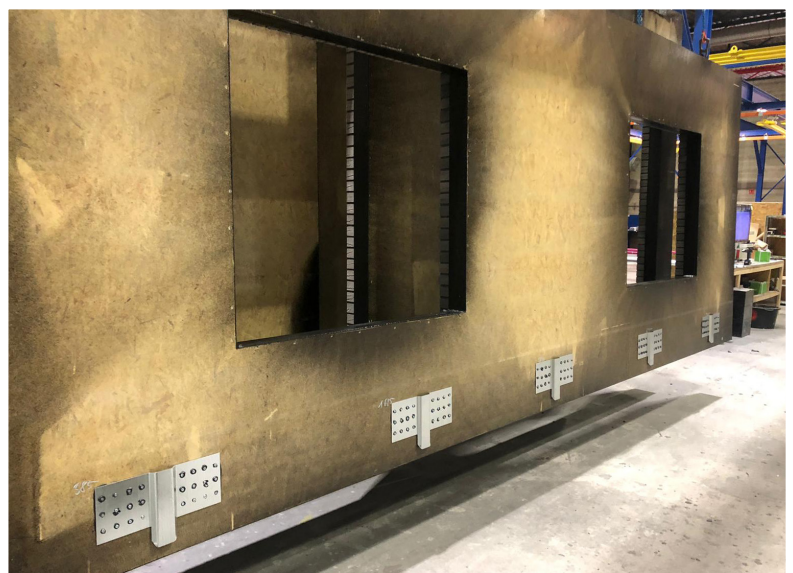
Figure 52 Anchors attached to the back of the panel
