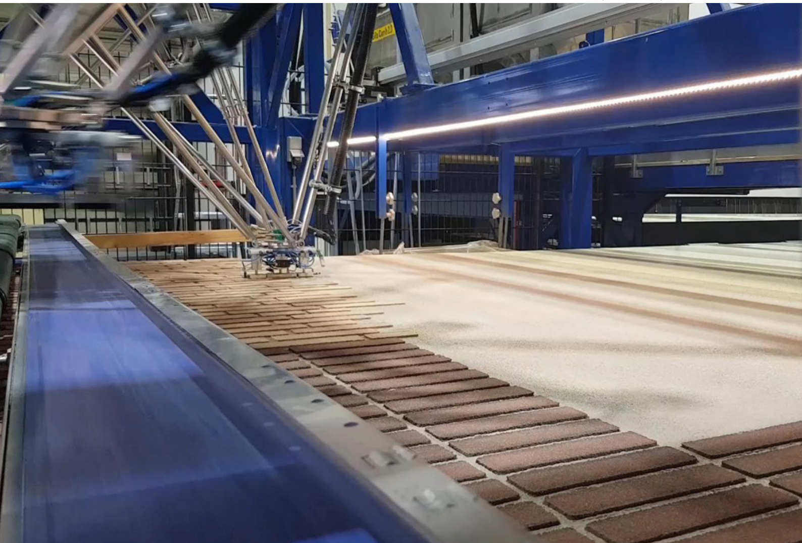
Figure 28 Automated mineral brick installation (picture by rcpanel.nl)
