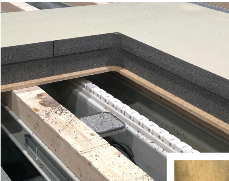
Figure 51 CNC cuts for openings
