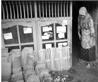
FIG.2.3 Bricks and tiles used to raise the floor.
