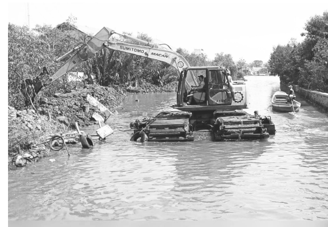
FIG.6.23 Excavator is cleaning up river sediment | Pekalongan river | 09.2020
