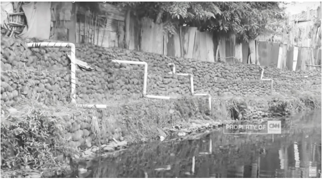
FIG.8.34 Wastewater is discharge into the river and the river is densely clocked by houses. Source: https://www.youtube.com/watch?v=VRpiViJcTRk&list=PLIjHHQqrlWu_tolzxp6N-iKrrheNNpup8&index=20
