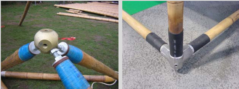
Figure 9.16: Connections with the bamboo stem with prefabricated standardized endings and steel connections; right connection developed by Sam van Veluw, left connection developed by the University of Aachen
