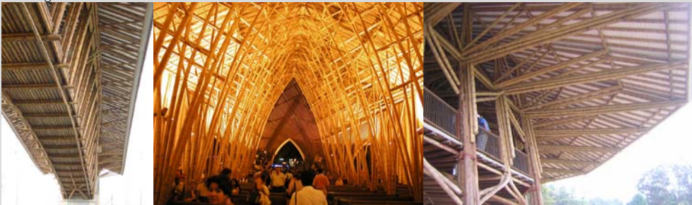
Figure 9.14: The strength of bamboo shown through various constructions in Colombia designed by Simon Vélez with spectacular eaves and spans
