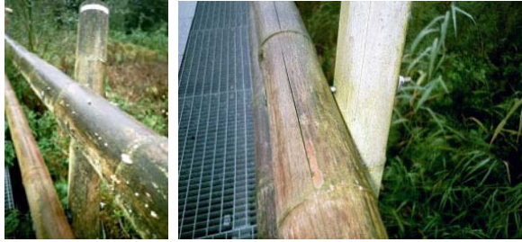
Figure 6.4: The bamboo stem is vulnerable to splitting and biological degradation when used outdoors, directly exposed to climatic circumstances (sun & rain)
