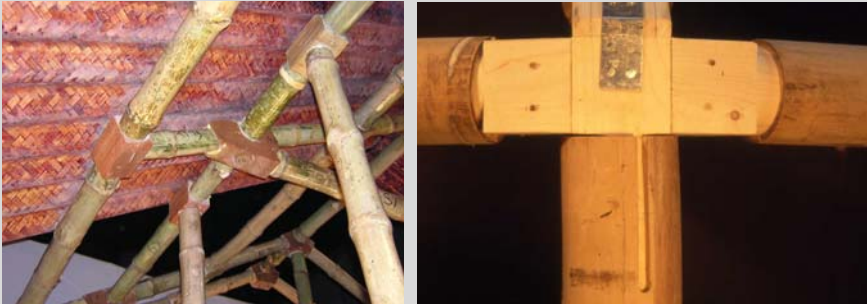
Figure 9.15: Connections with the bamboo stem based using wooden props facilitating easier connections; left connection by Bambu Tec, right connection by Oscar Ace
