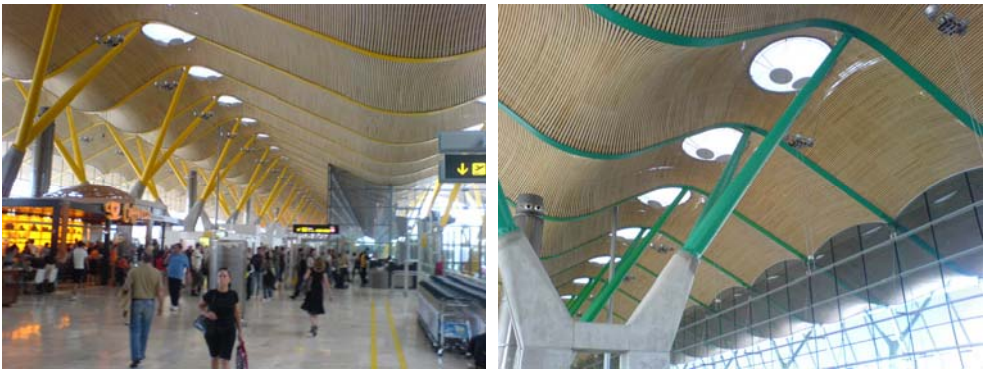
Figure 9.18: Curved plybamboo laths used in the ceiling of the new airport in Madrid designed by Richard Rogers
