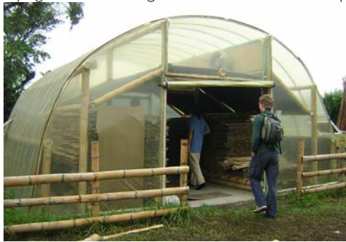
Figure 5.3: Low cost solar powered drying chamber for bamboo strips in Colombia developed by Jörg Stamm
