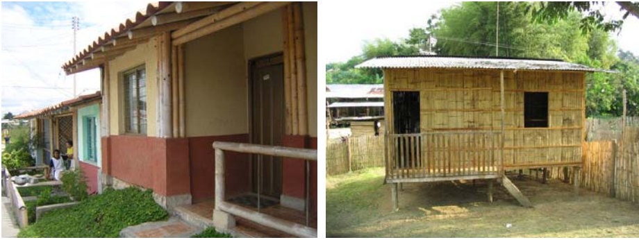
Figure 5.36: Low cost bamboo housing in Latin America
