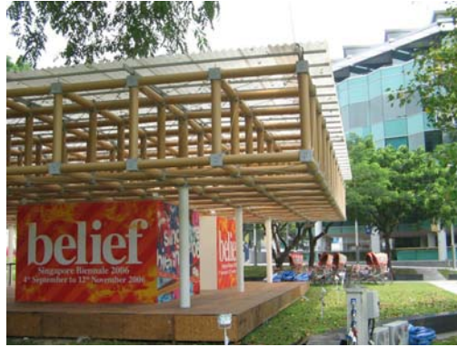
Figure 9.1: Cardboard is slowly being adopted in the building industry, especially in temporary buildings (e.g. pavilions)
