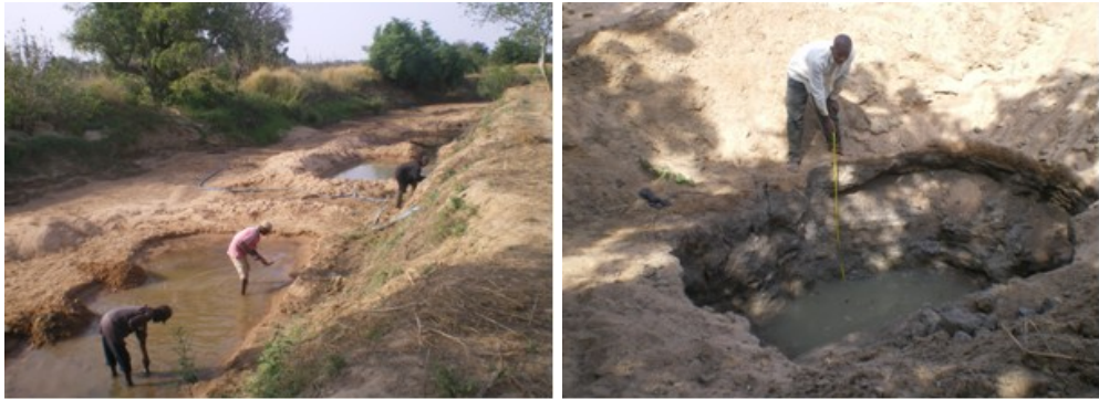
Figure 5.7: a) Initial stages of Riverine Alluvial Dugouts b) Latter stages of Riverine Alluvial Dugouts.
