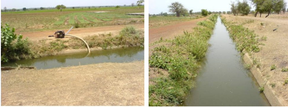
Figure 4.5: a) Pumping water from main canal in Vea b) Main canal transporting water by gravity to the fields in Vea
