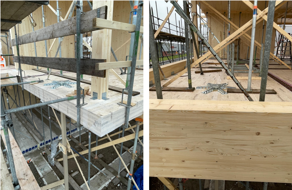
Figure J.3: Spider connection
