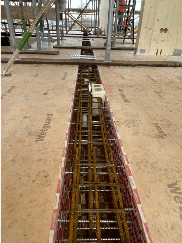
Figure J.4: TC Fusion connection
