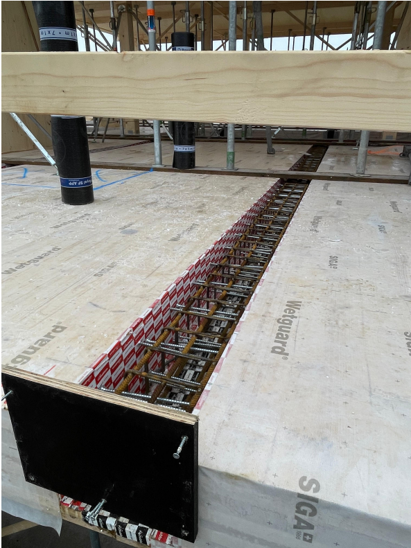
Figure J.4: TC Fusion connection
