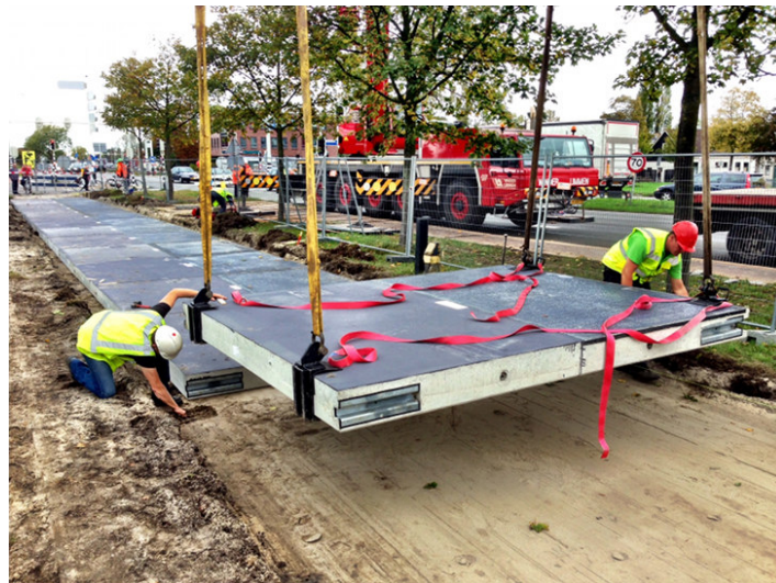
Figure 6-15: TNO SolaRoad installation. Image Source: [14]
