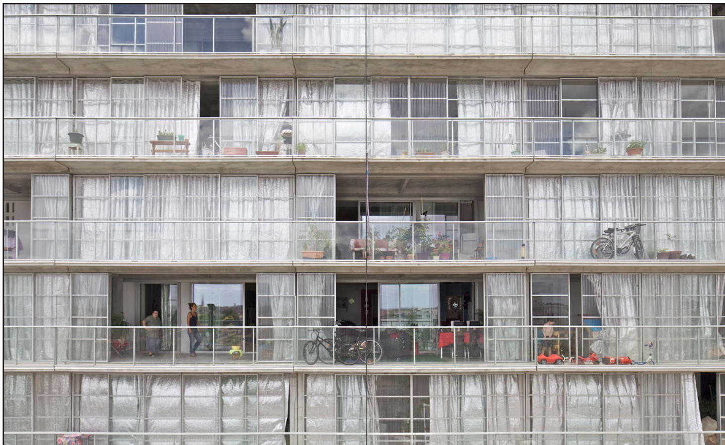
Inner facade south-west: Grand Parc, Lacaton & Vassal architectes
